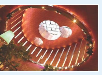
All lighting armatures, ballast units, cables, as well as the basic construction itself must be invisible from the public point of view, which is 9 metres below the construction. Prolyte has developed an ellipse shaped truss construction of 25 x 17 metres, which can be completely covered with sandwich panels, which can be painted in any wanted colour.
